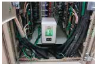
▲ Water purification plant facilities (Bupyeong, Incheon)
