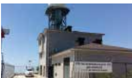
Turkey Meteorological Radar Station
