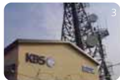
1. Perimeter Surveillance System for the President Office, 2. Royal Tombs of the Joseon Dynasty-UNESCO World Heritage with total integrated surveillance system (include CCTV) 3. KBS Digital TV Relay Station
