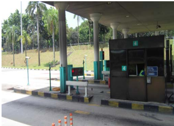
Toll gate Booth
