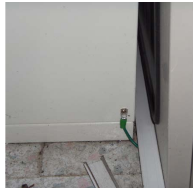
Auto fire extinguisher bonding
