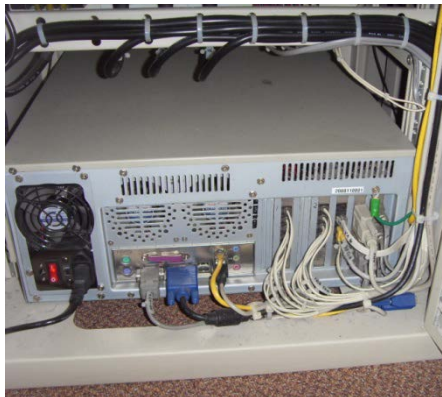
Grounding Bonding improvement
