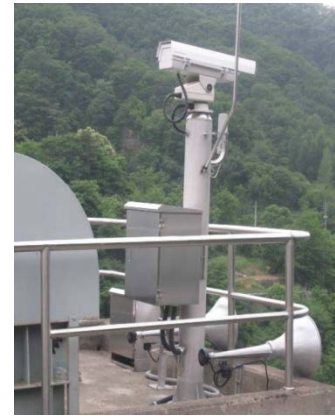
Downstream monitoring CCTV & eca3G
