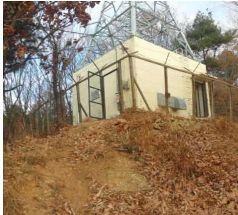
Relay station Tower
