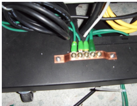
Rack Ground Bar installation
