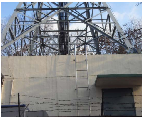
Relay station Tower
