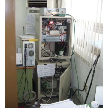
Comm Protector installation
