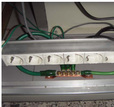
Rack Ground Bar installation
