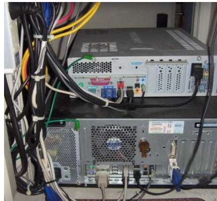
Grounding Bonding improvement
