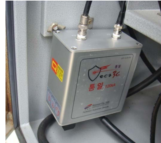
Communication Support Troop - CCTV system protection
