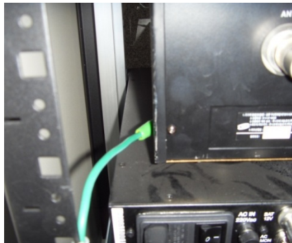
VHF Equipment Bonding improvement
