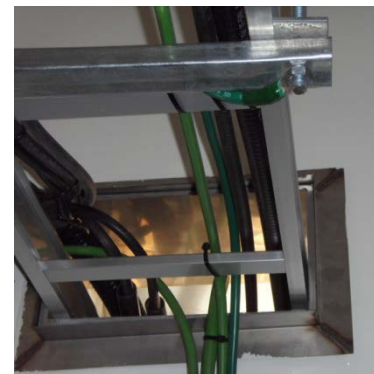
Cable Tray Bonding
