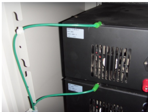
VHF Equipment Bonding improvement
