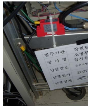
Comm Protector installation
