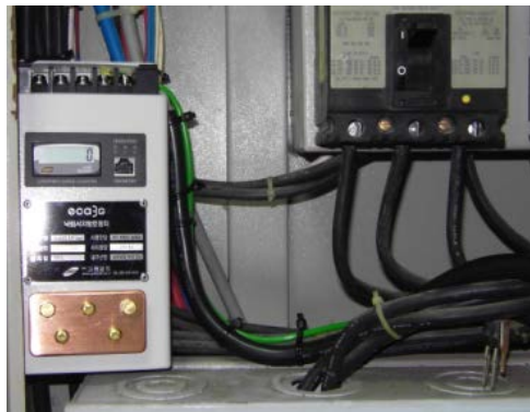
<eca3G > positioning in DB
