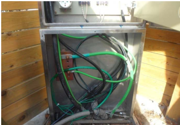
Equi-potential Bonding
