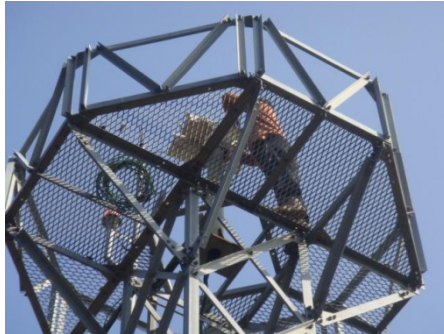
CCTV Tower bonding
