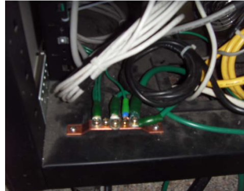
Rack Ground Bar installation
