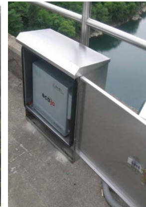
Downstream monitoring CCTV & eca3G
